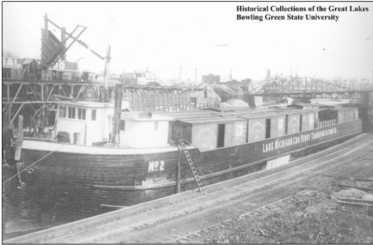
Figure 1 - The Railroad Car Ferry Number 2 in Operation (used with permission[2])
