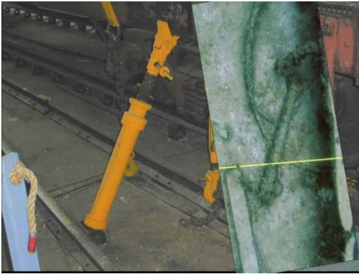
Screw Jack ( In Use on L, In Situ on R )
